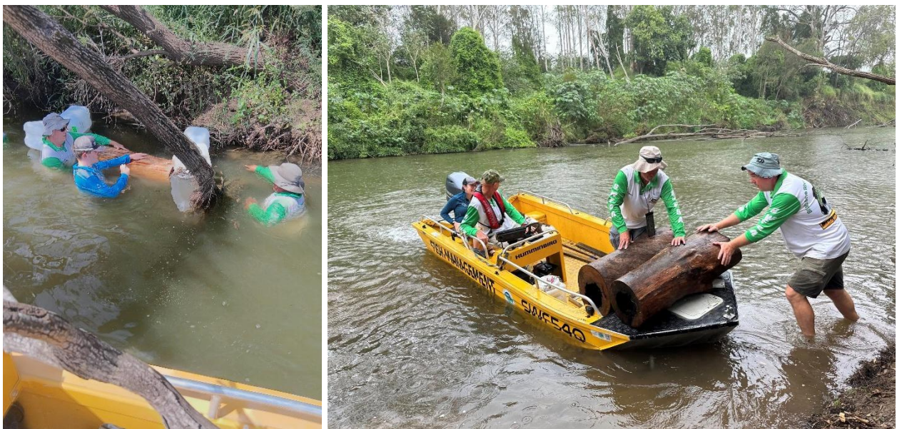
Float Swim method Vs Boat method to move logs into place.
