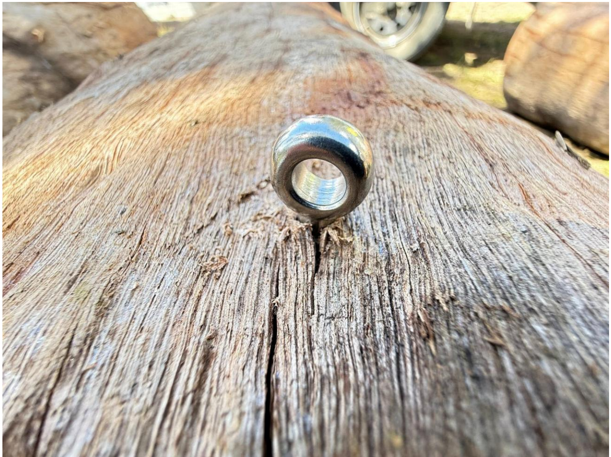
Stainless steel eye bolts were screwed into the logs to secure in place with gal chain.
