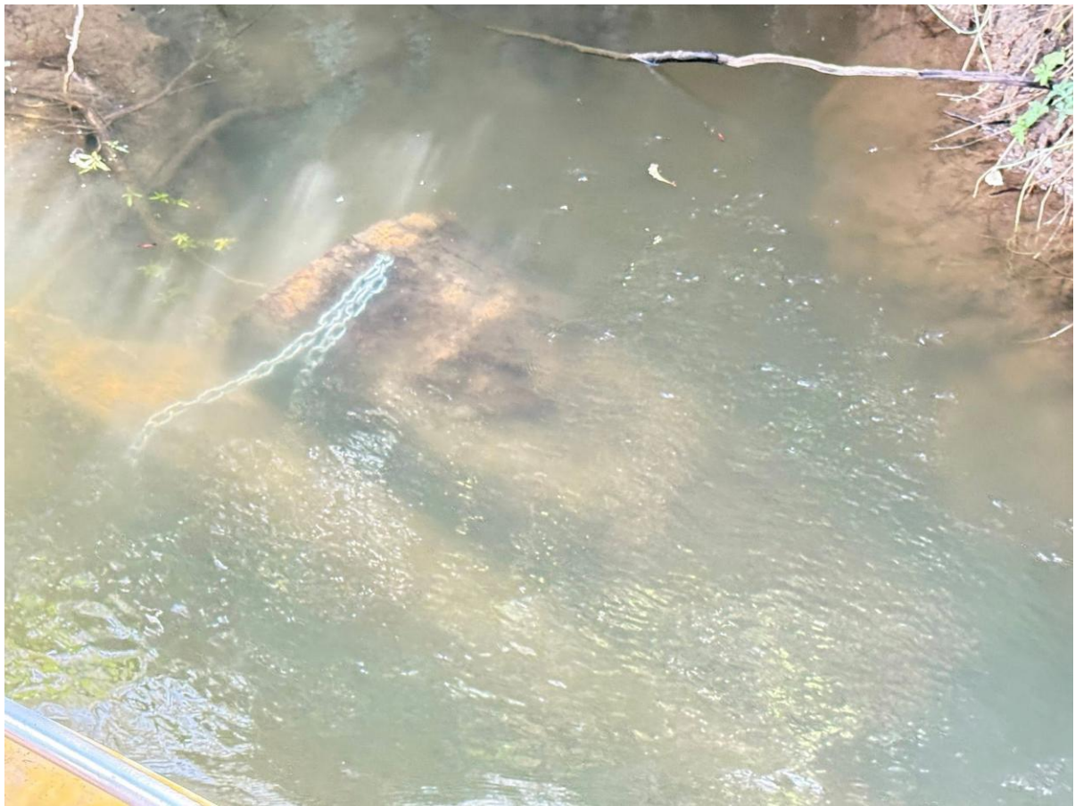
Stainless steel eye bolts were screwed into the logs to secure in place with gal chain.
